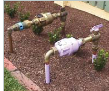
FIGURE 3 - RECYCLED WATER AND DRINKING WATER METER ASSEMBLIES
