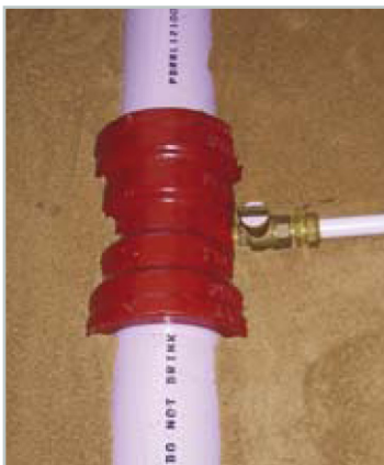
FIGURE 2 - RECYCLED WATER MAIN AND PROPERTY SERVICE
